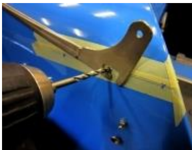
fig.3 Drilling the hole in the side of the body
